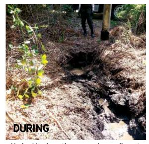
Hydro-Vac in action removing sediments
