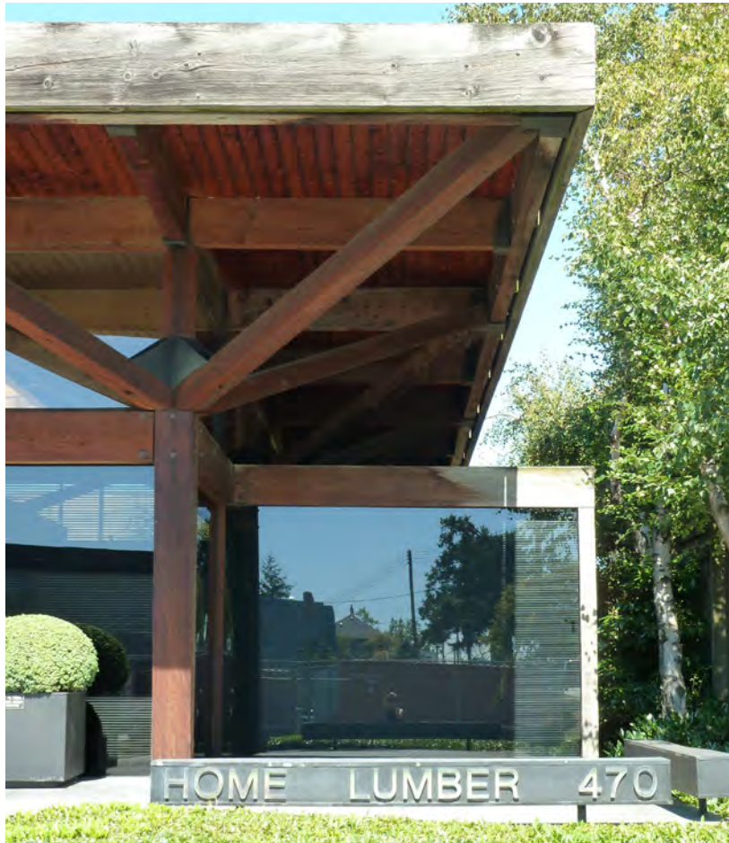
Home Lumber Office - 470 Ardorsier Road
