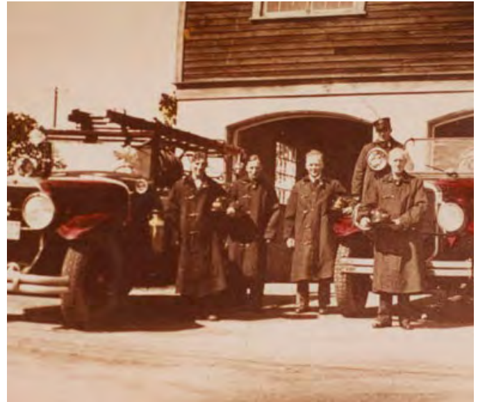
Fire Hall No. 1, 1939.
