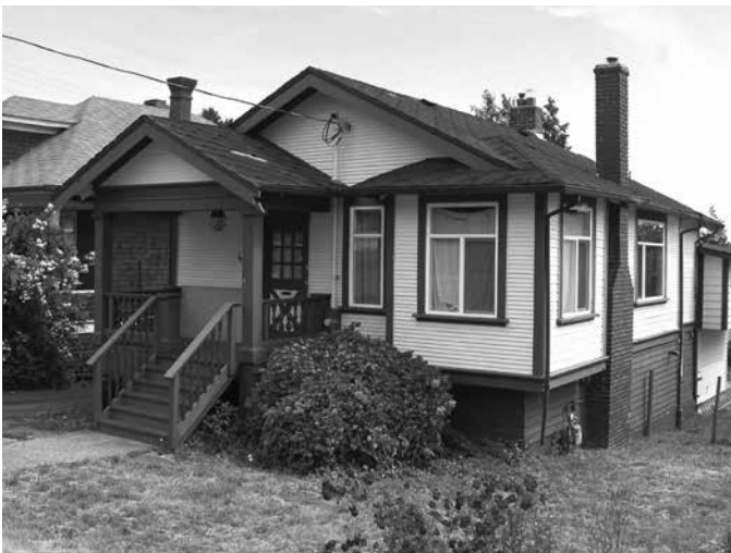
Tapscott Residence, 415 Boleskine Road.
