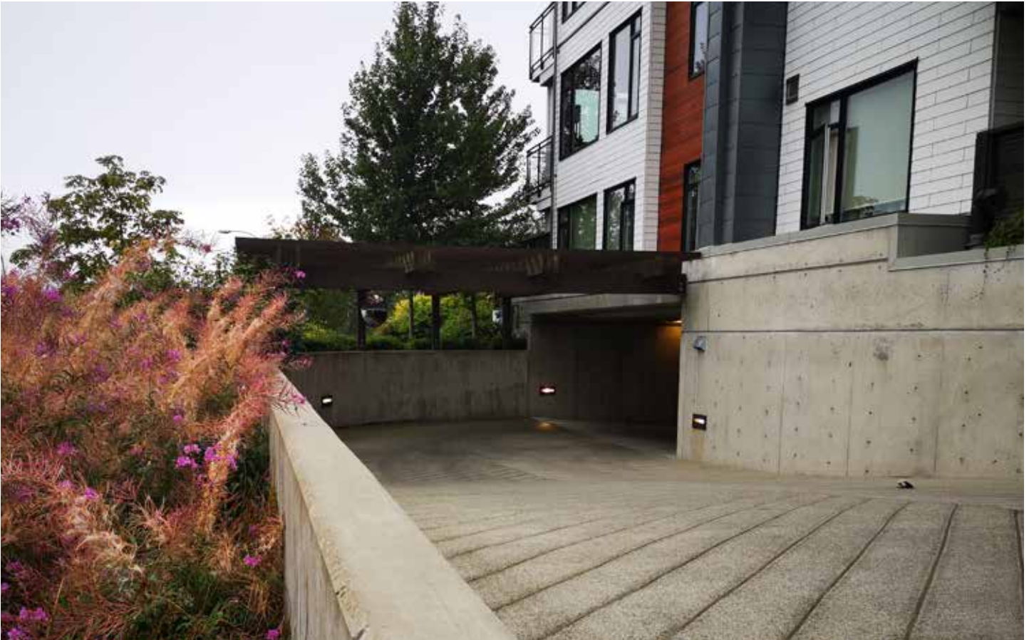
Underground parking off Huxley Street
