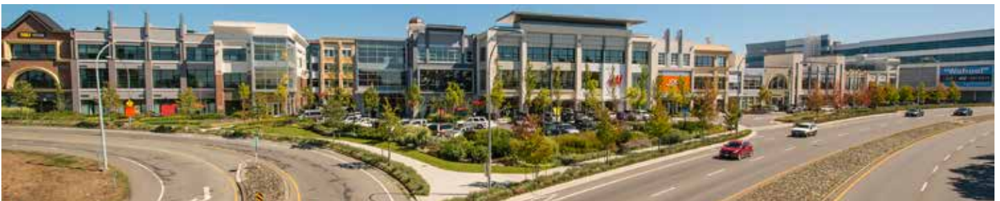
Douglas Street at Carey Road
