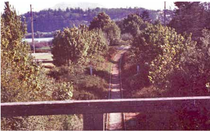
Bridge crossing over CNR Rail (now Lochside Regional Trail), 1971.
