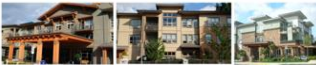
3 Storey Apartments u/g parking
