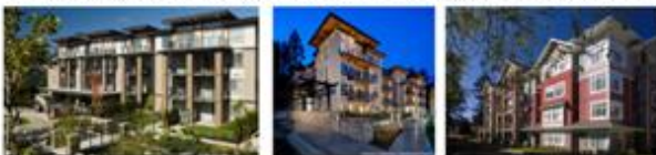
4 Storey Apartments u/g parking
