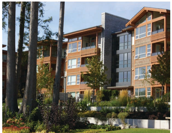
Figure 6: Design features and building materials contribute to the richness of place
