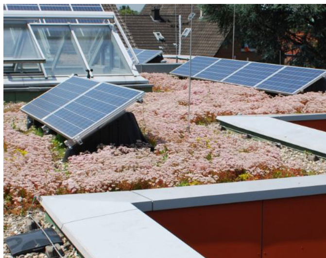
Figure 15: Flat roofs are opportunities for amenity areas, renewable energy generation, and green roofs
