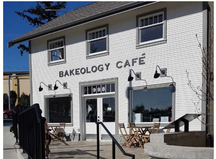
Figure 12: Downcast exterior lighting reduces light pollution
