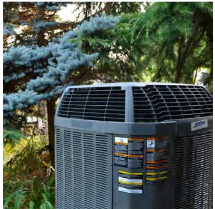
Electric heat pump
