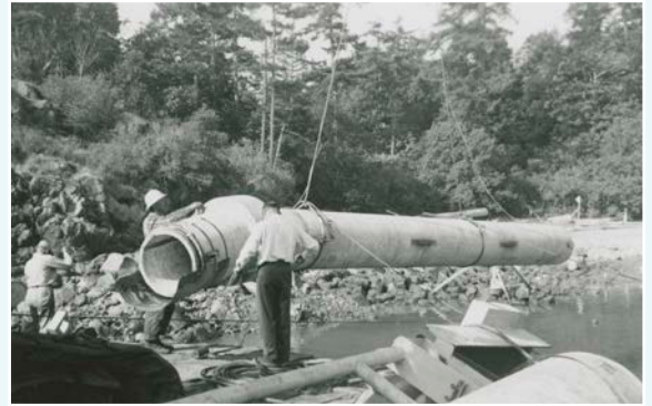
1980-015-258c Construction of Arbutus Outfall 1955
