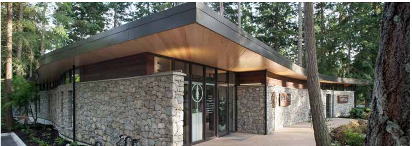
Figure 10.7: Encourage the use of quality building materials and finishes
