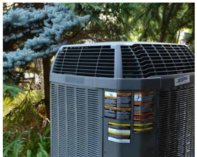
Electric heat pump
