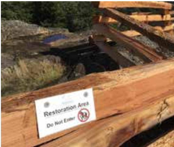
Finished fence with Restoration Area sign
