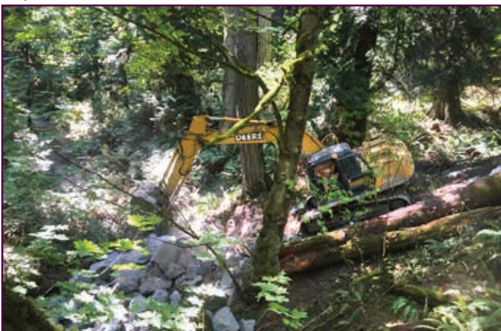
Rock delivery at Ash Bridge.
