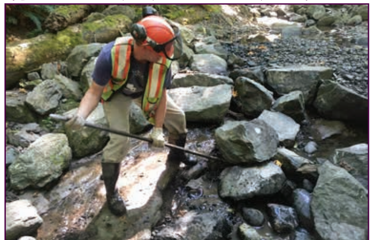
Boulder placement along stream bed.
