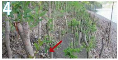
**Photograph 3 and 4.** Dense live staking can be used where erosion is causing a problem. The dense pattern of the live stakes slows the flow velocity of the river and allows sediment to be deposited (red arrow).
