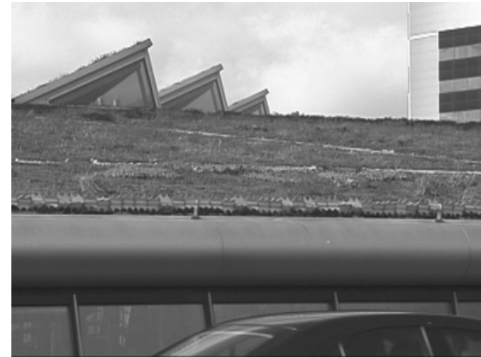
Figure 7-23 Lightweight Extensive Green Roof
