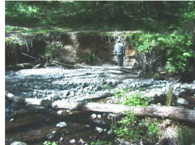
Figure 1-6 Channel Down-Cutting (due to increased volume)
