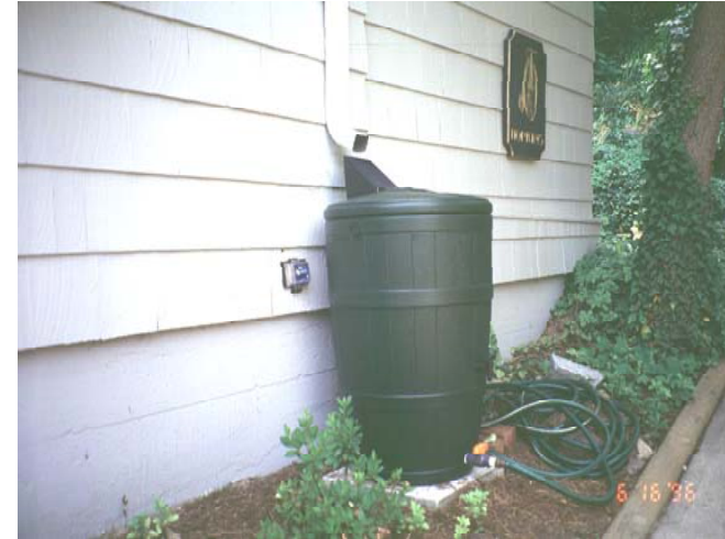
Figure 7-28a Rainwater Re-use using Rain Barrels
