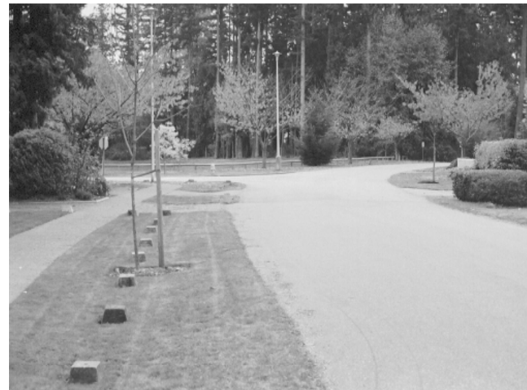
Figure 7-10 Infiltration Swale Along Roadway
