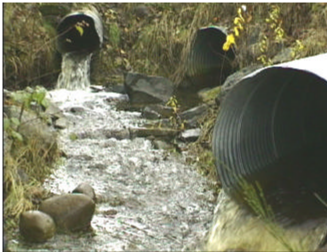
Figure 1-5 Multiple Drainage Culvert Installations
