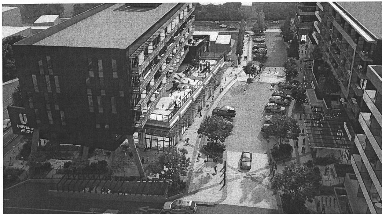
Figure 9: Plaza Between Buildings D & B (looking south) (provided by WA Architects)
