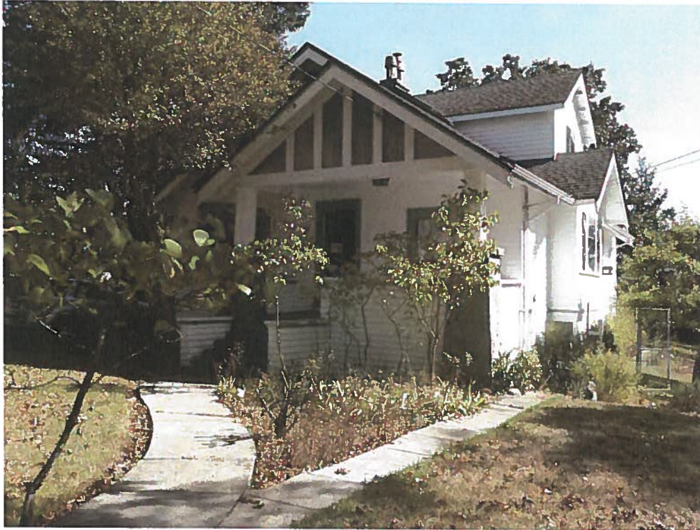
Photo: 3905 Hobbs St. Front (North) Elevation
