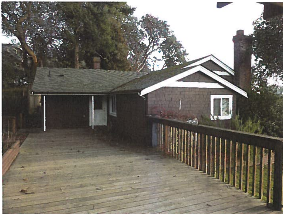
Looking southeast towards the cottage
