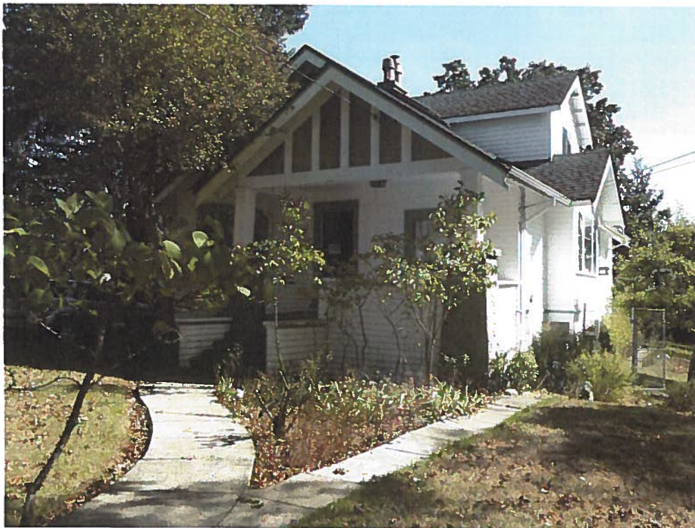
Photo: 3905 Hobbs St. Front (North) Elevation
