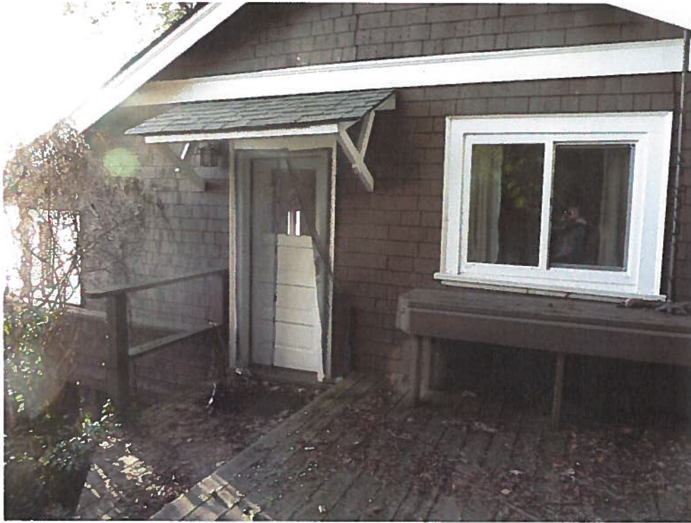
Looking north towards the cabin
