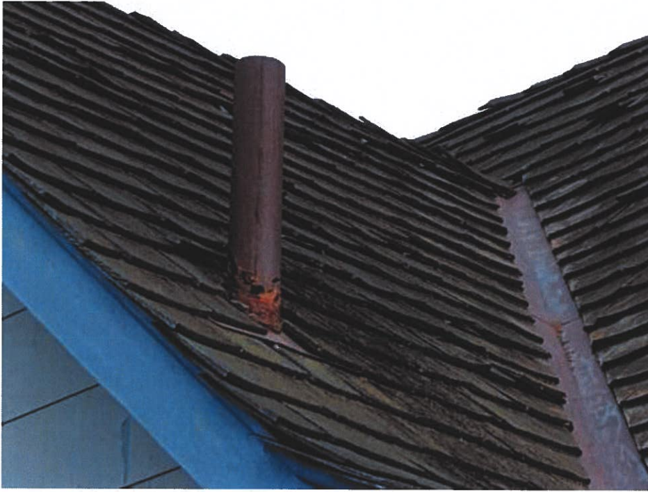
Picture of the existing roof, including metal flashing
