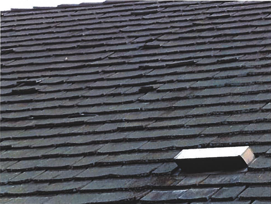
Picture of the existing roof
