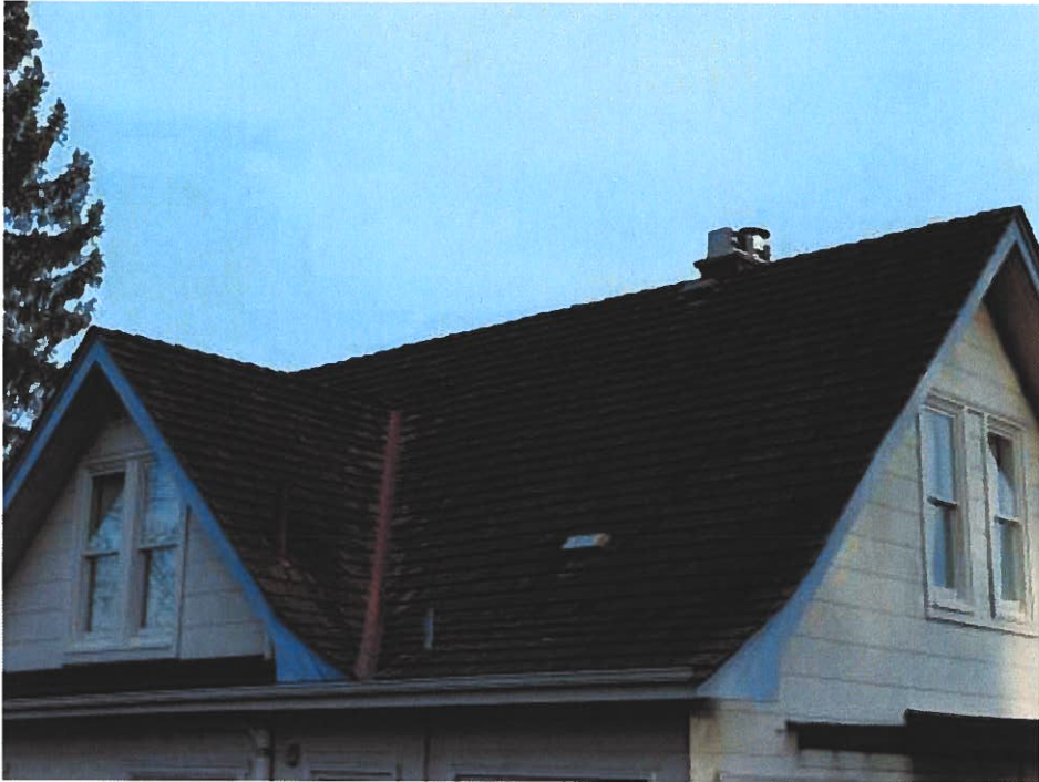
Picture of the existing roof
