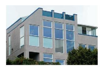
These windows are exposed to wind-driven rain. Water resistant products and installation methods must be used.
