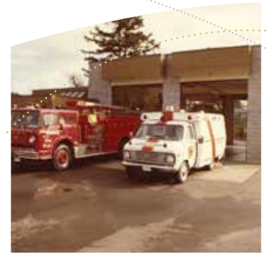
Fire Hall 2 shortly after its construction as it appeared in 1978. 1
