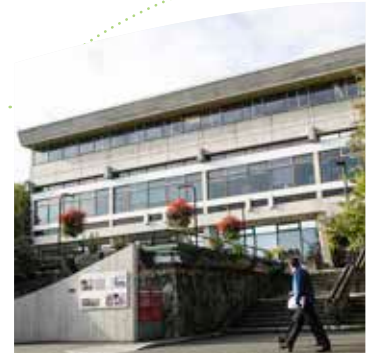
Municipal Hall East entry.
