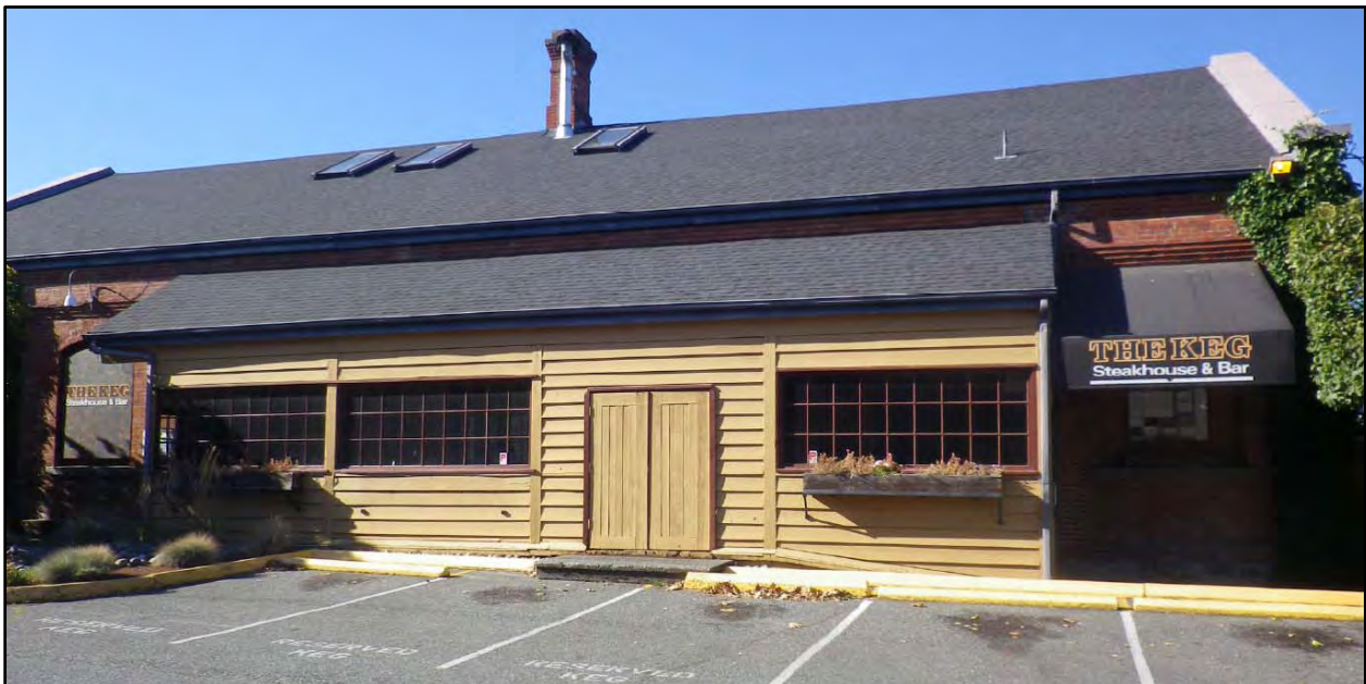
Figure 3: Existing Entrance Vestibule
