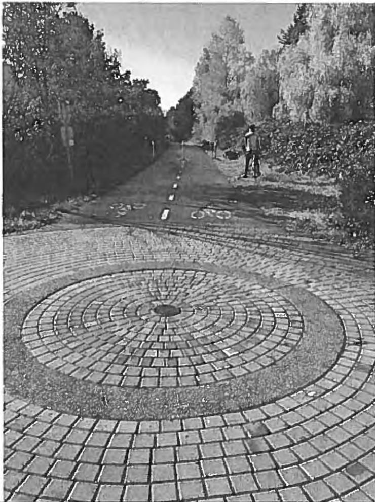
Lochside at McKenzie and Borden. Why have any bollards here?
