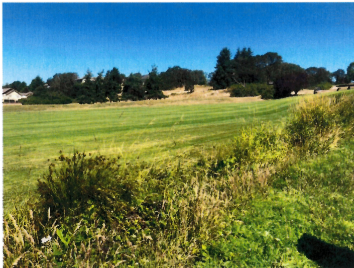
Photo 8: Creek channel at the outlet of storm drain adjacent to 7 th Hole fairway
