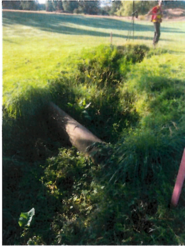
Photo 1: Creek channel upstream of 4 th Hole Fairway. Note steel water main crossing the creek.
