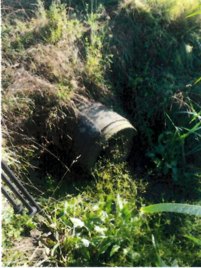
Photo 7: Outlet of storm drain under 7 th Hole fairway
