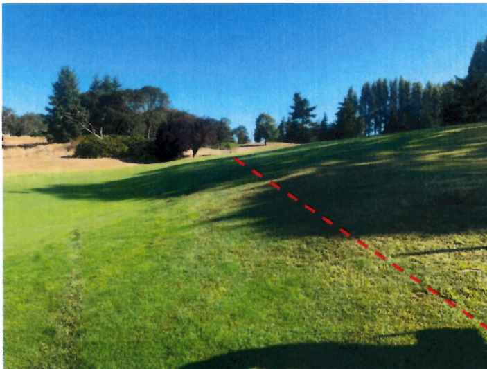
Photo 6: Alignment of storm drain to the south of 7 th Hole green. Red dashed line shows approximate alignment.
