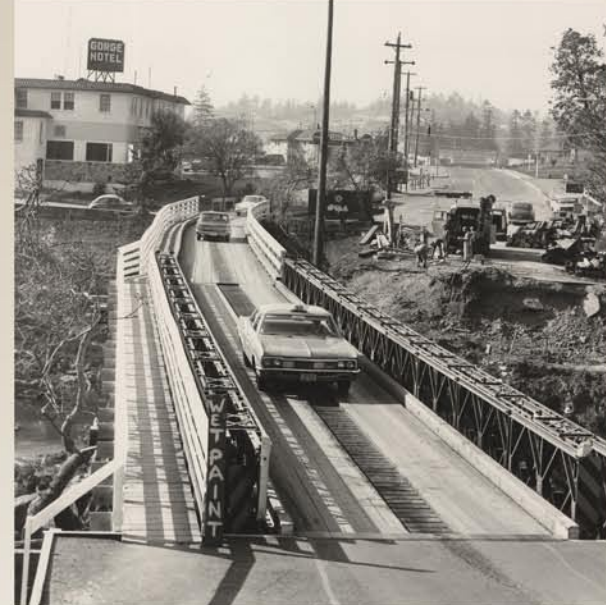
A temporary crossing during the construction of current bridge with view of the Gorge Hotel to the south, circa 1966/67. Courtesy of Saanich Archives, 1987-003-002.
