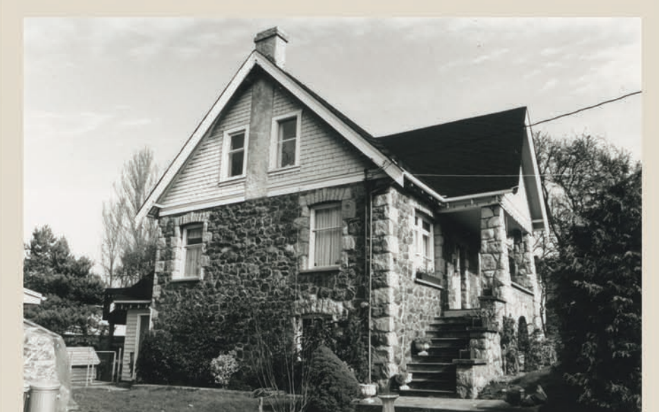
1744 Kisber Avenue, photo circa 1987-90. Courtesy of Saanich Archives, 2006-015-239a. This stone house was built during WWI (1914-18) by master stonemason Donald Montgomery who, having bought the stone from the blasting site of the Provincial Normal School, (now Camosun College on Lansdowne), hauled it back load by load in a wheelbarrow!
