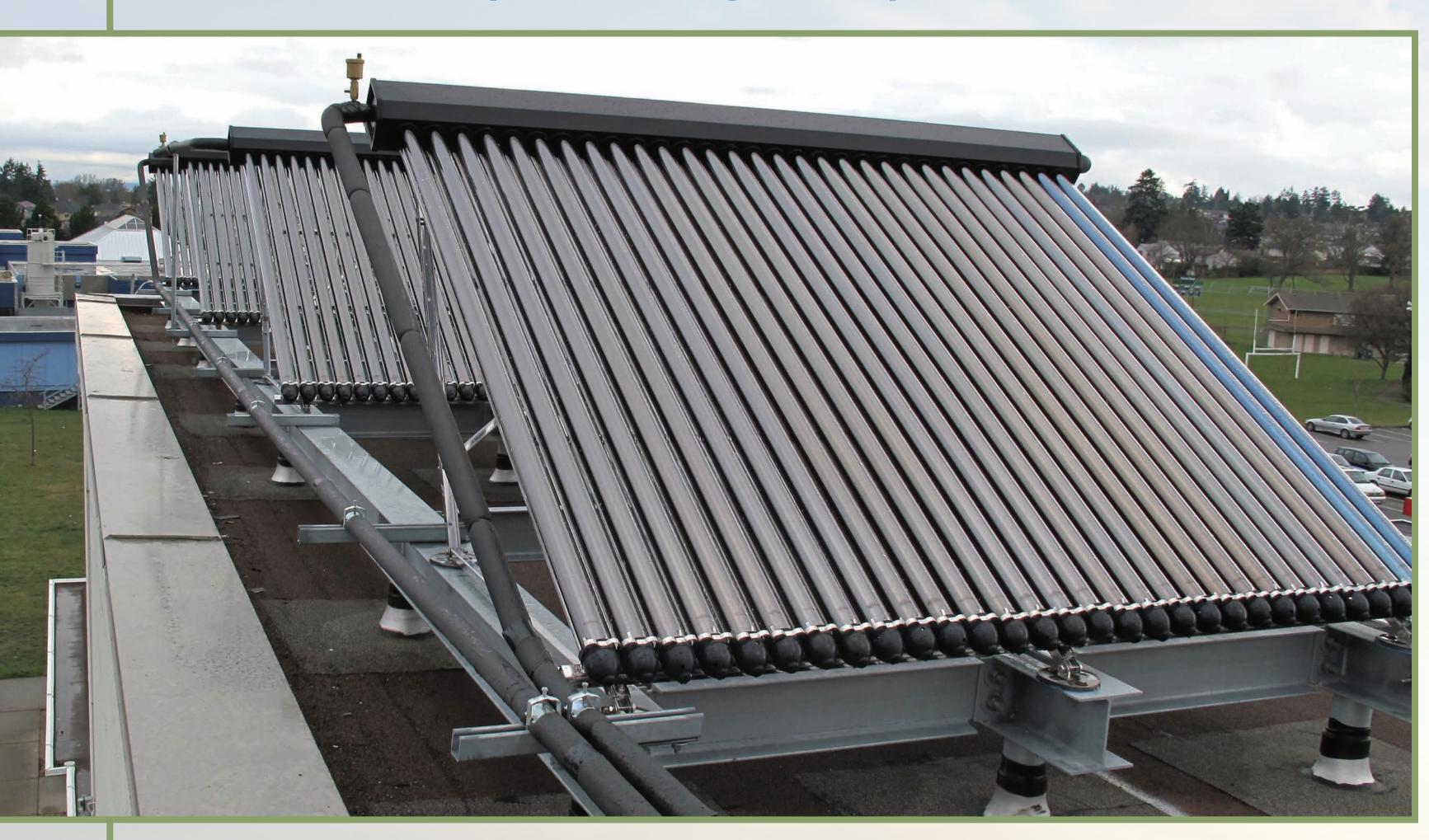
Look up on the roof to see the four panels that are now providing heat to the Centre's shower water. By using a renewable energy source the system will reduce our carbon footprint by 20 tonnes annually.
