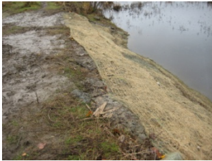
Erosion Control near Storage Barn, December 2012
