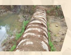
At this location, Wray Creek was once enclosed in an old wooden culvert dating back to approximately 1968. The pipe was failing and it was decided to "daylight" the creek by removing it from the pipe and restoring habitat.
