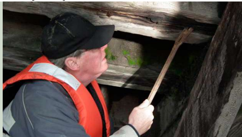
Photo: Craigflower Bridge condition assessment
