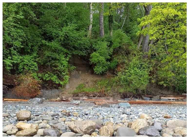
Photo 2: Slope toe failure at Station 9+45 (taken 24 April 2024).
