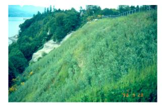
Photograph 1 and 2. Wattle fences were used to treat the Quadra sediments of the Point Grey cliffs. The average in-situ slope is 70°. Growth of the pioneering species used to construct the wattle fences started a successional processes that will see these slopes vegetated forever.
