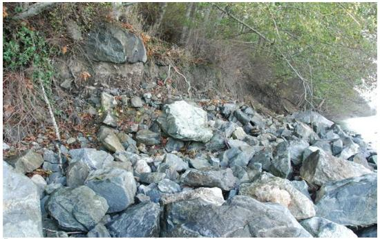
FAILURE OF THE RIP-RAP REVETMENT AT MOUNT DOUGLAS PARK HAS ALLOWED CONTINUED EROSION OF THE SHORELINE.
