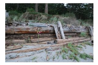
**Photograph 5 & 6.** Rotting log walls can be used to protect shorelines where the foreshore rises steeply from the beach. This system shoreline protection system has been in place for many years.
