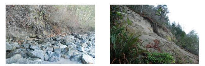
Photograph 1 & 2. Failure of the rip-rap shore protection (left) has allowed continued erosion of the toe of the Quadra sediment slope (right). This has resulted in slumping of the slope.
