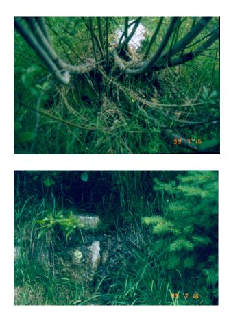
Photograph 5, 6 and 7. Live pole drains provide drainage immediately and one year after installation (left). They continue to drain the slope 14 years after installation (right upper and lower) as well as creating habitat for later successional species to invade (right lower).
