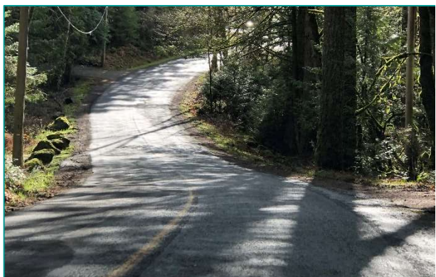
Photo 1 – Horizontal and Vertical Curve
